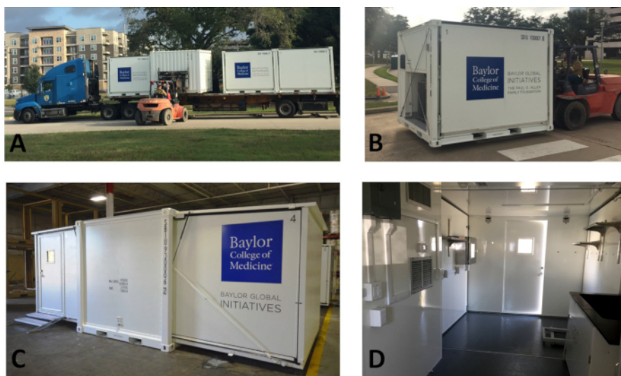
Figure 1. Laboratory facility prototype. (A, B) Transport mode; (C) Deployed mode: outside; (D) Deployed mode: interior. Please click here to view a larger version of this figure.
